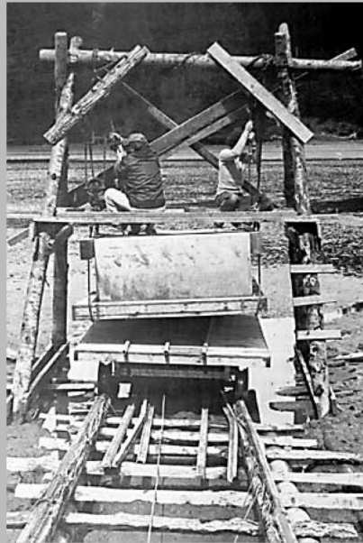
Fig. 20. At those times when the tide was out, an A-frame was used to hoist a completed float off of the railway carriage. Then the carriage was removed and the float was lowered onto the tidal flat. After the tide came in the float was towed out to join the growing flotilla. The two individuals are Don Baxter and Tom Butler-Cole (Courtesy Richard Larson)
