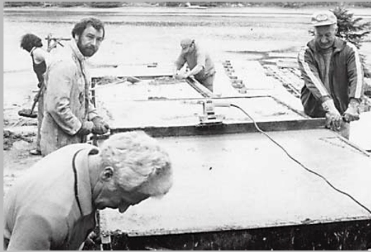
Fig. 9. Levelling the surface using a screed rail, prior to rifting. Figures, clockwise, are Peter McMillan, Don Baxter, Tom Butler-Cole, Cliff Carey and Bob Hanson (Courtesy Richard Larson)
